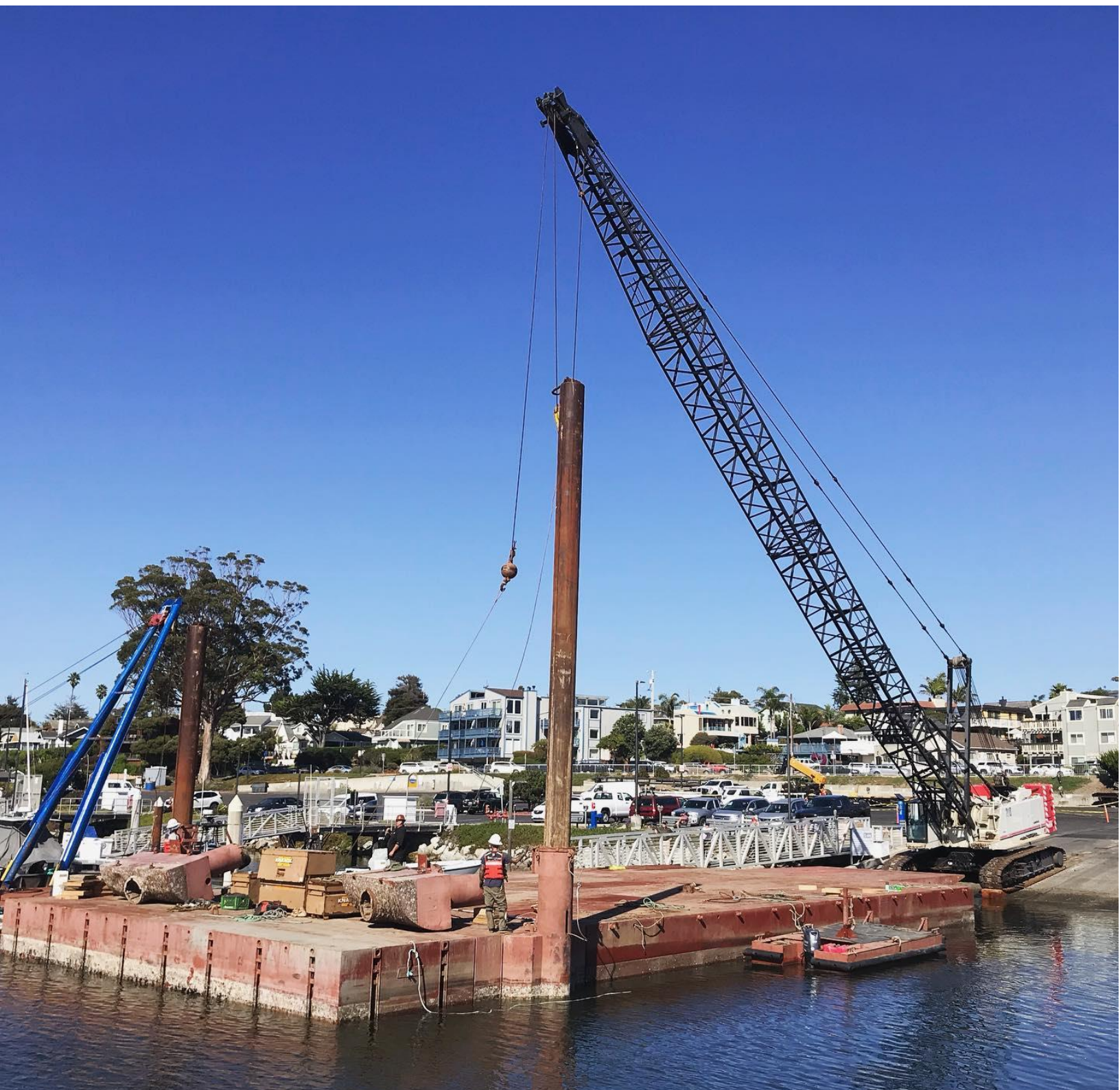
Figure 8-4: Aldo's Seawall Project
