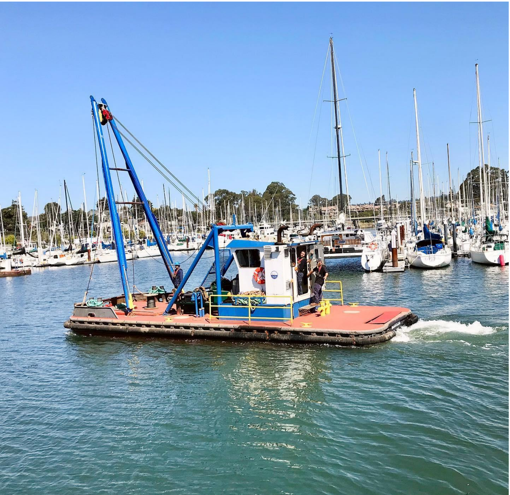
Figure 8-6: SCPD Dredging Operations.
